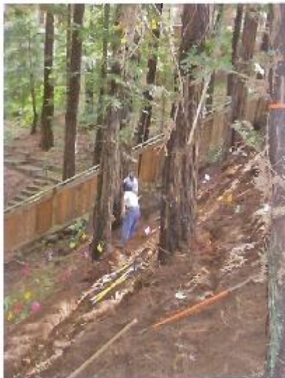
A steep slope installation in California — 65% slope.
